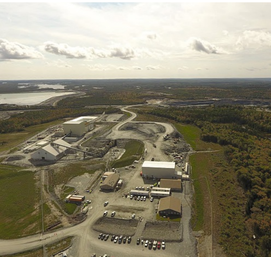
Dig here: St Barbara's operations at Moose River in Nova Scotia
